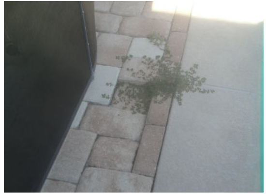
brick pavers settling
