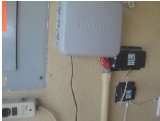
conduit loose at control panel and wall
