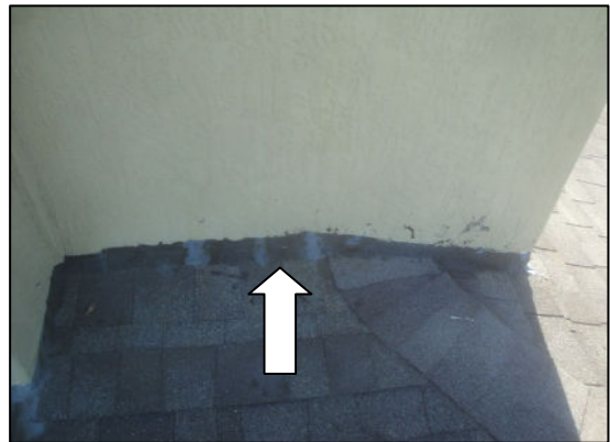
tarred in flashing
