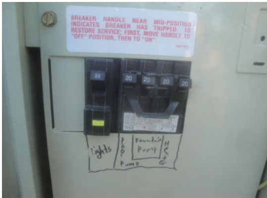
pool heater not on separate breaker
