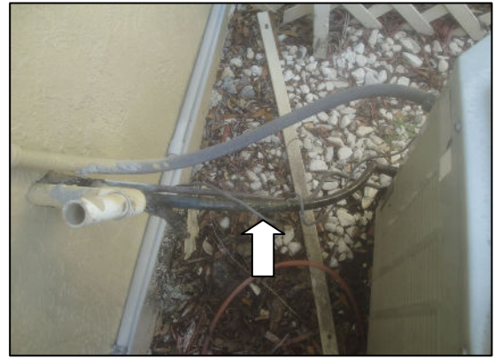
missing suction line insulation
