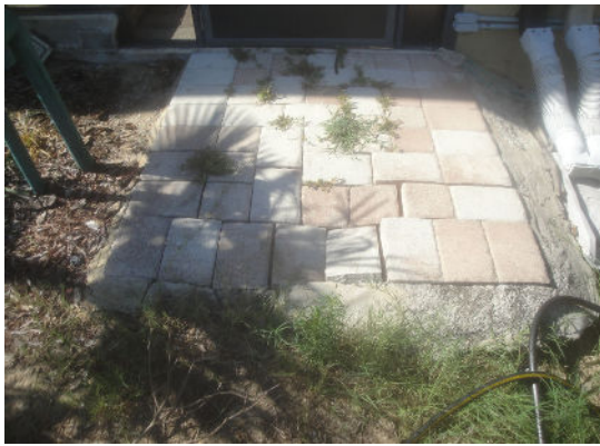
brick pavers settling
