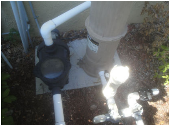
leaky seal at pump
