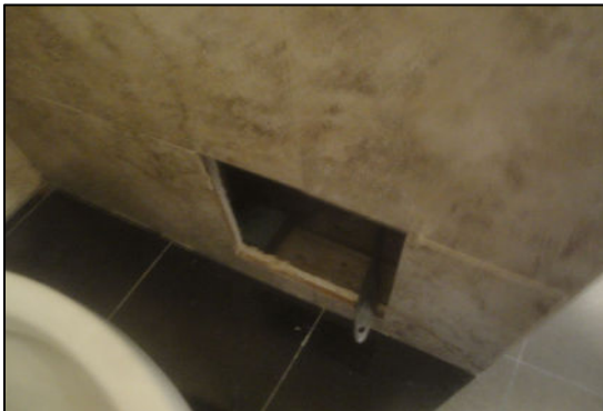
missing acces cover panel
