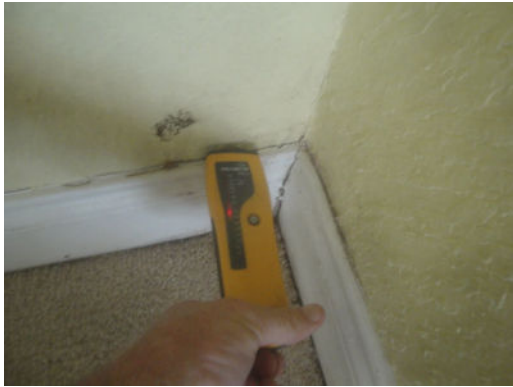
water intrusion/mold
